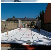
(left) The Supergrund foundation system features three layers of EPS 100 insulation, with the bottom layer shown here with joints taped, and foam filling around service penetrations; (below left) The taped second layer of EPS, before channels are cut to contain heat recovery ducts and then the top layer of 100mm EPS laid over; (below), installation almost complete of the reinforced steel mesh for the concrete slab, with underfloor heating also installed.
