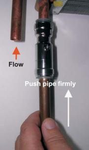
and push the flow pipe in as far as the end stop in the quick connect. Repeat for return. Open the in line valves. Connect the three core cable, and that's it.
